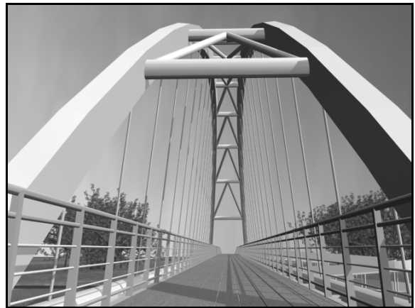
Figure 8: Central span path view.
