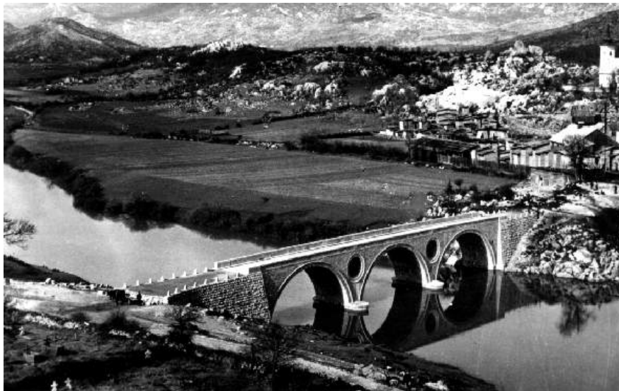
Figure 2. Lika Bridge in Kosinj – a supreme example of excellent aesthetics (author: Frković).
