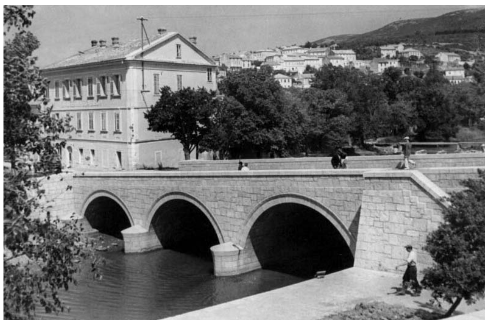
Figure 7. Dubračina bridge in Crikvenica.
