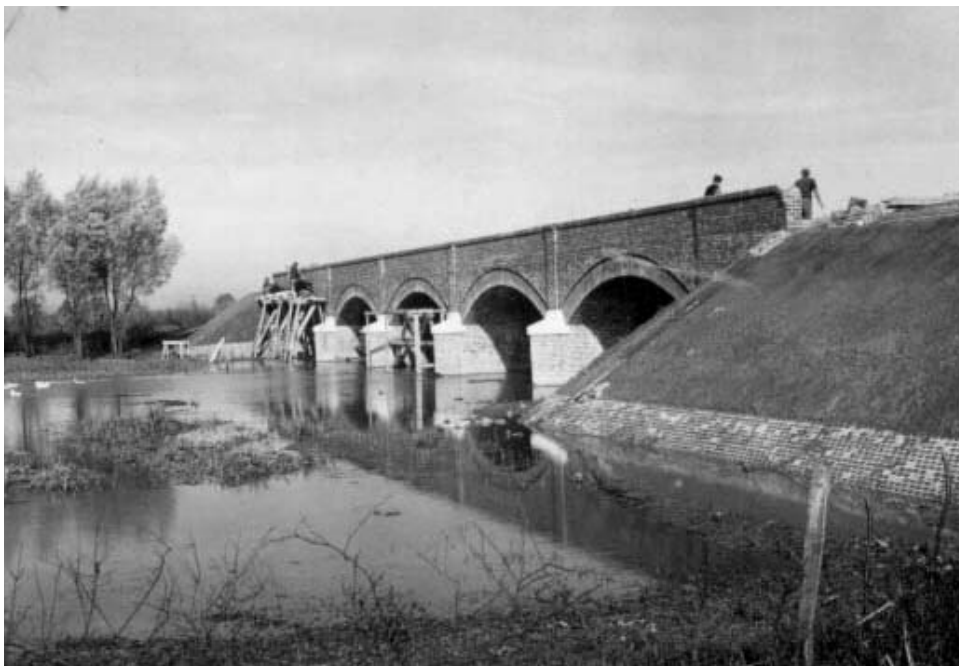
Figure 5. Vuka river bridge in Ernestinovo.
