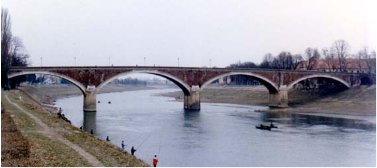
Figure 3. Kupa Bridge (Sisak) constructed by Frković.
