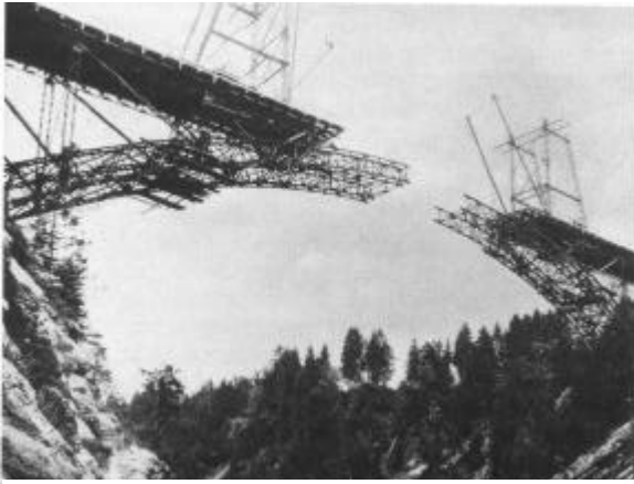
Figure 8 Ammer shuttering, Echelsbach, Austria
