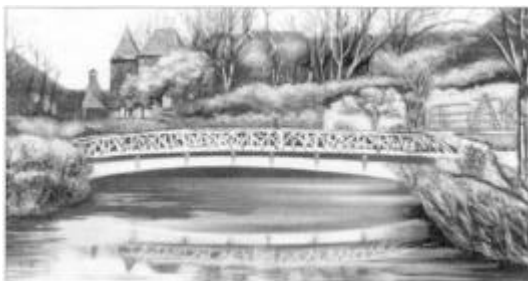
Figure 5 Tilière de Chatelet Arch Bridge
