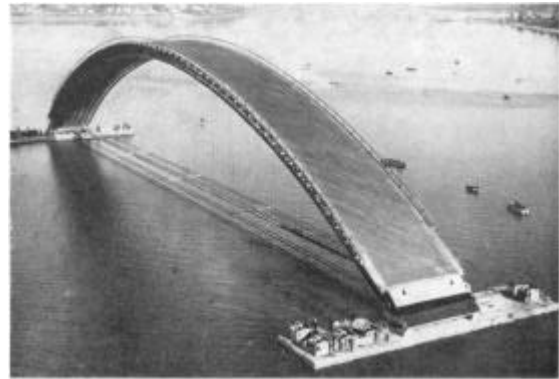
Figure 9 Plougastel arch shuttering
