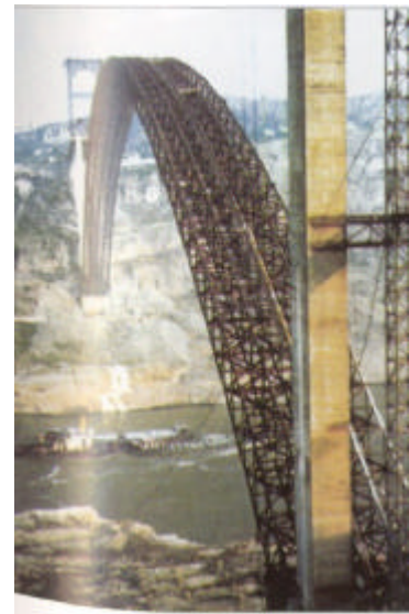
Figure 15 Waxian Shuttering
