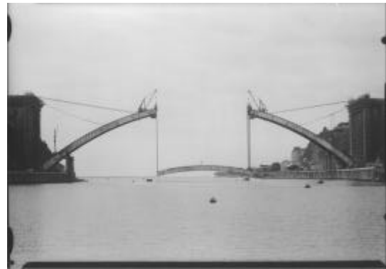
Figure 11 Lifting Arrabida central shuttering
