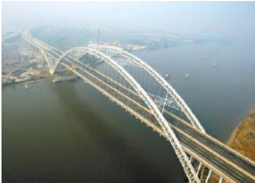
Figure 26 Yajisha arch, Zhugian river China
