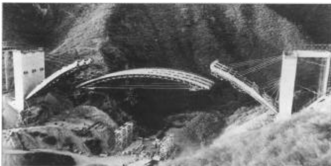
Figure 10 The Guaira arches shuttering, Venezuela
