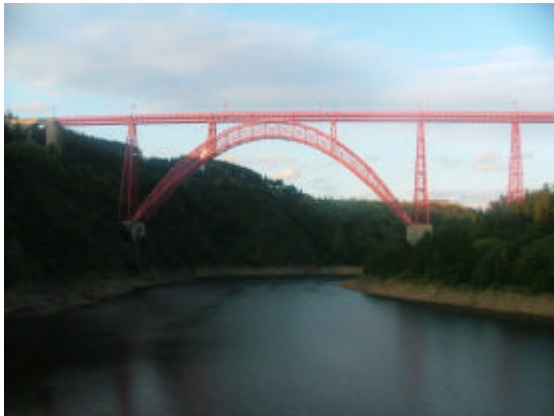
Figure 3 Garabit Viaduct, France
