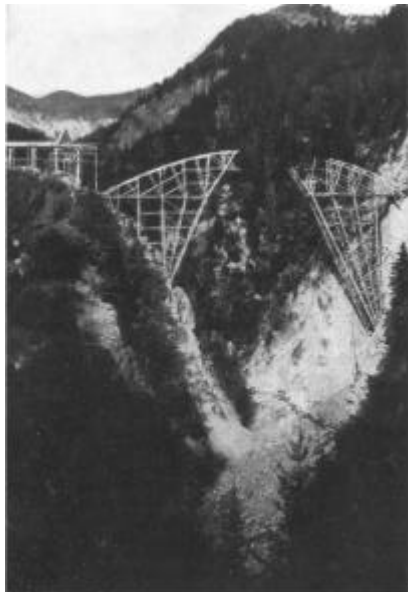
Figure 7 Sanginatobel Shuttering
