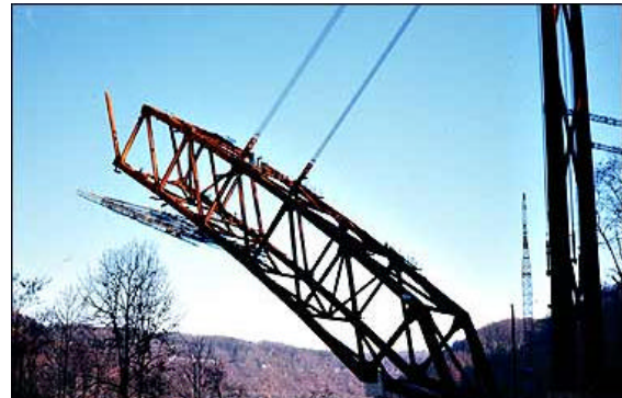
Figure 21 New Gorge River Arch construction
