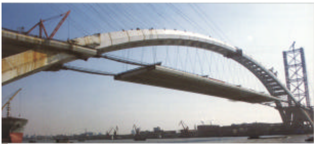
Figure 23 Lifting Deck, Stays and horizontal cables
