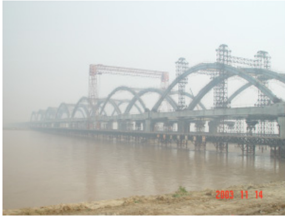
Fig. 6 Side view of temporary bridges
