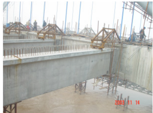
Fig. 9 Installation of cross beams
