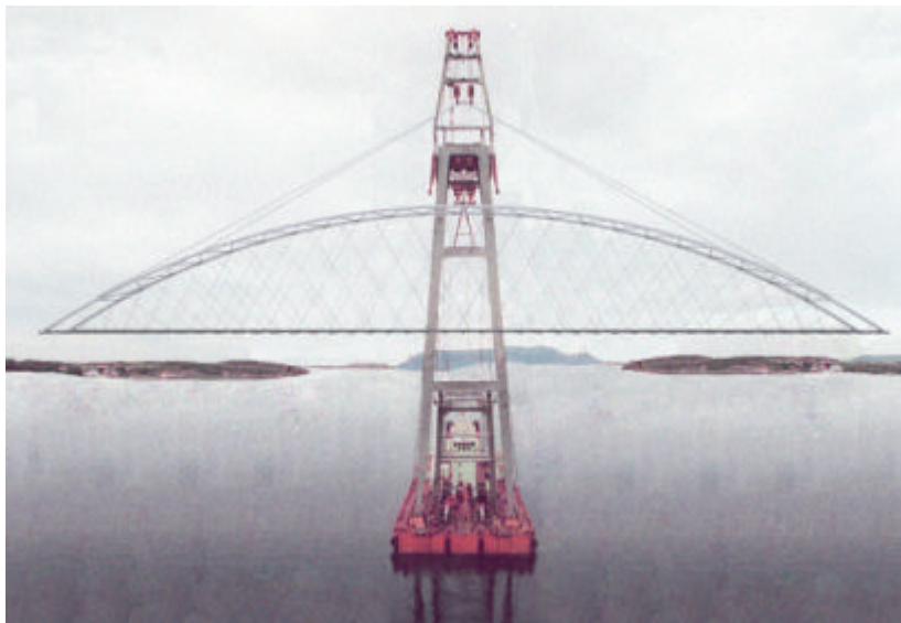
Fig. 10. Lifting of the steel skeleton of the bridge in fig. 6
