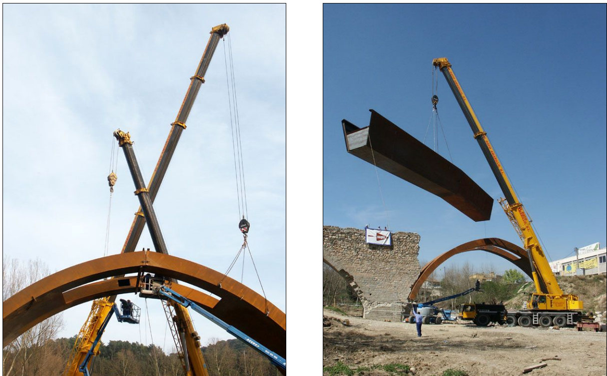
Figure 8 – Erection of the arch and lifting of the deck
