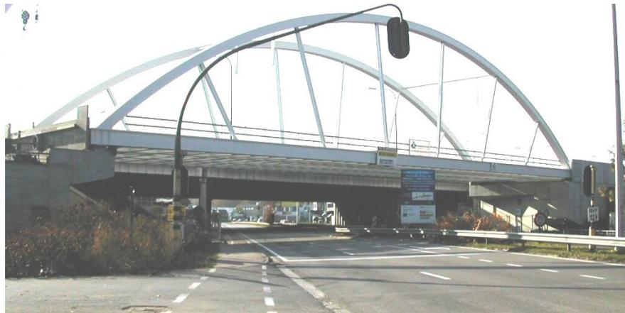
Fig 6 : Fan arranged hanger system
