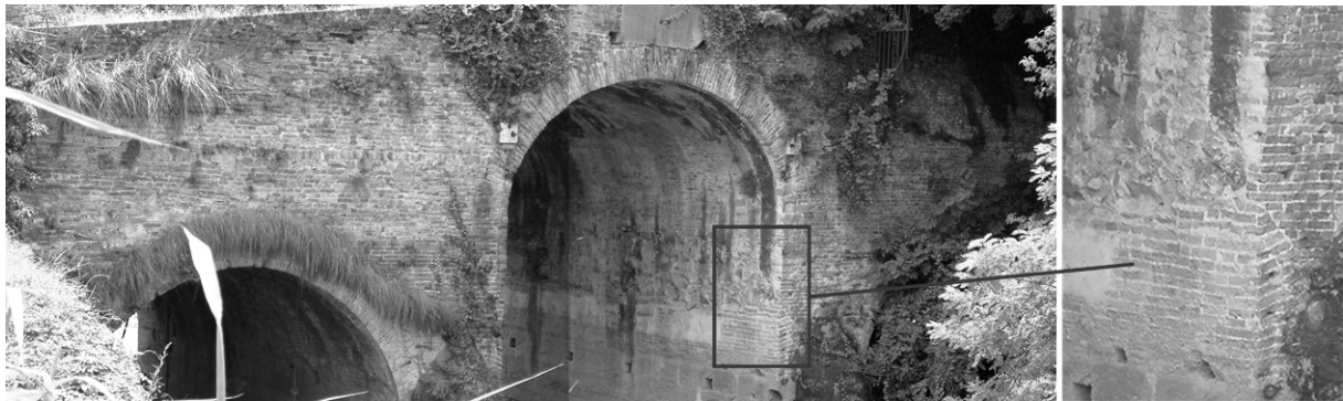
Figure 7: The central barrel with a detail of the abutment of the ancient vault
