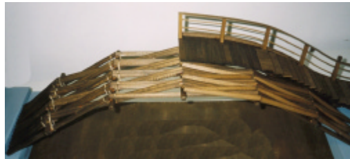
Figure 12: Timber model of Rainbow Bridge.
